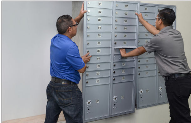
Figure 15 – Butt each unit's trim up against the other.
