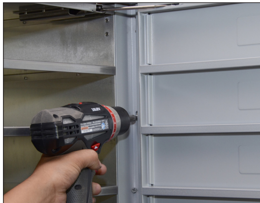
Figure 16– Secure units together using connector machine screws
